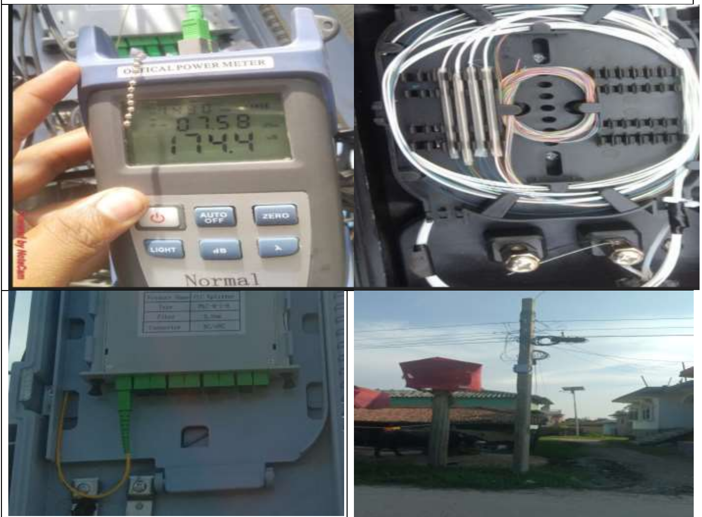
Some Glimpse during preventive / corrective actions carried out
